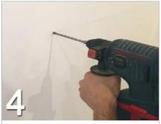
Use a masonry drill to drill first with 6/7 mm and finish with a 10mm bit. Drill to a depth of 70mm max.
