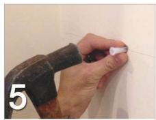
Insert the 10mm rawl plugs provided and if required use the hammer to ensure the plugs are flush.
