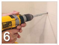
Use a cordless drill to drive in the 12 mm shelf support all the way leaving just enough for some adjustment.
