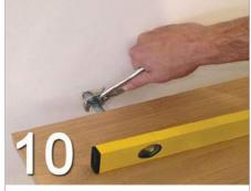
Using the spirit level and spanner (or pipe grips) gently rotate the shelf support left/right until level.
