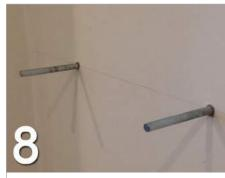
Place a spirit level across each of the supports once installed and check all for level and 90 degrees.
