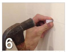
Insert the 7mm rawl plugs provided and if required use the hammer to ensure the plugs are flush.
