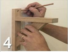
Now mark on the wall for each bracket hole (for modern brackets allow for the keyhole when marking out)
