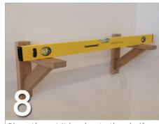
Place the spirit level onto the shelf and check for level, make any adjustments by tapping the brackets before fastening screws tight.
