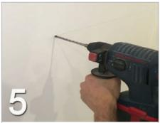
Use the masonry drill with a 7mm masonry or SDS bit, and drill to a depth of 75mm, (you can use masking tape as a depth guage)
