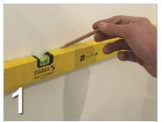
Use the spirit level to mark a level line at the required point of installation.
