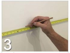
Transfer measurements across to the line on the wall for each centre point.
