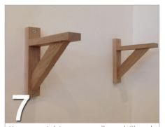
Use a pozi driver or cordless drill and fix each bracket to the wall just hand tight for now using wall screws
