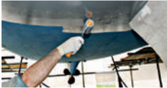
Apply Hempel's High Protect with roller
