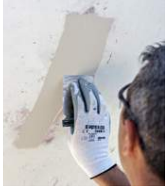
Fairing any defects
