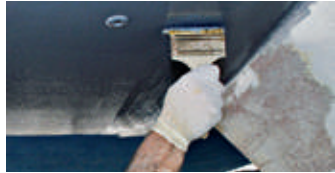
Lay off Hempel's High Protect in opposite direction with brush
