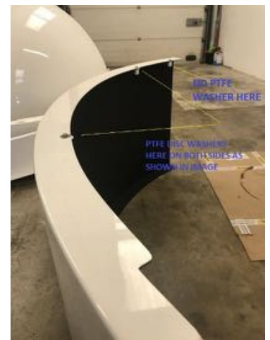
2.7 roller setup showing position of the PTFE washers.
