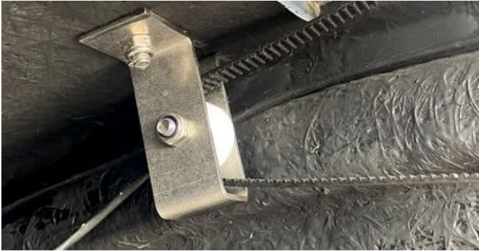
Rear bracket shown with shutter fully open
