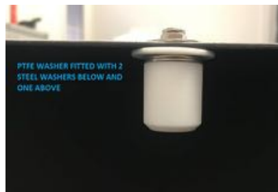
2.7 roller setup showing position of the PTFE washers.
